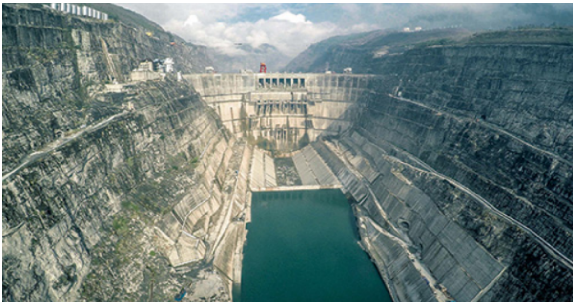
Figure 2: A Photograph Showing the Rogun Dam Project Under Construction
